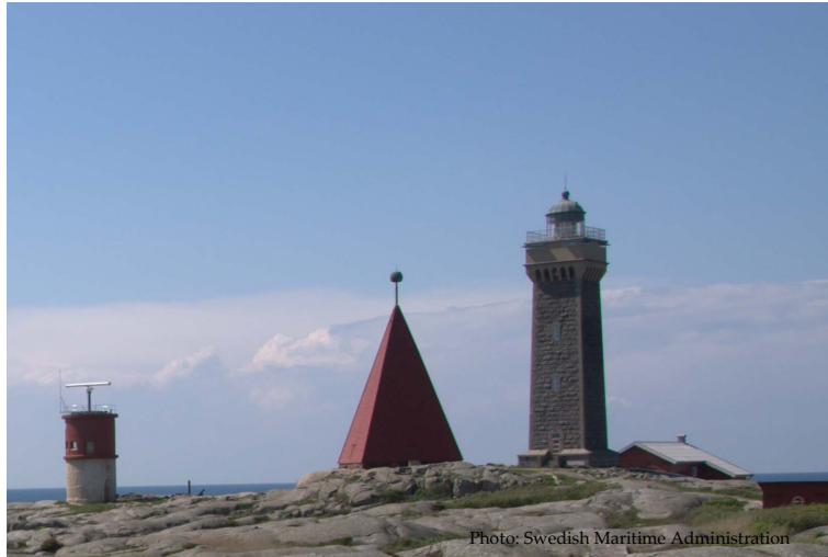
Photo: Swedish Maritime Administration
