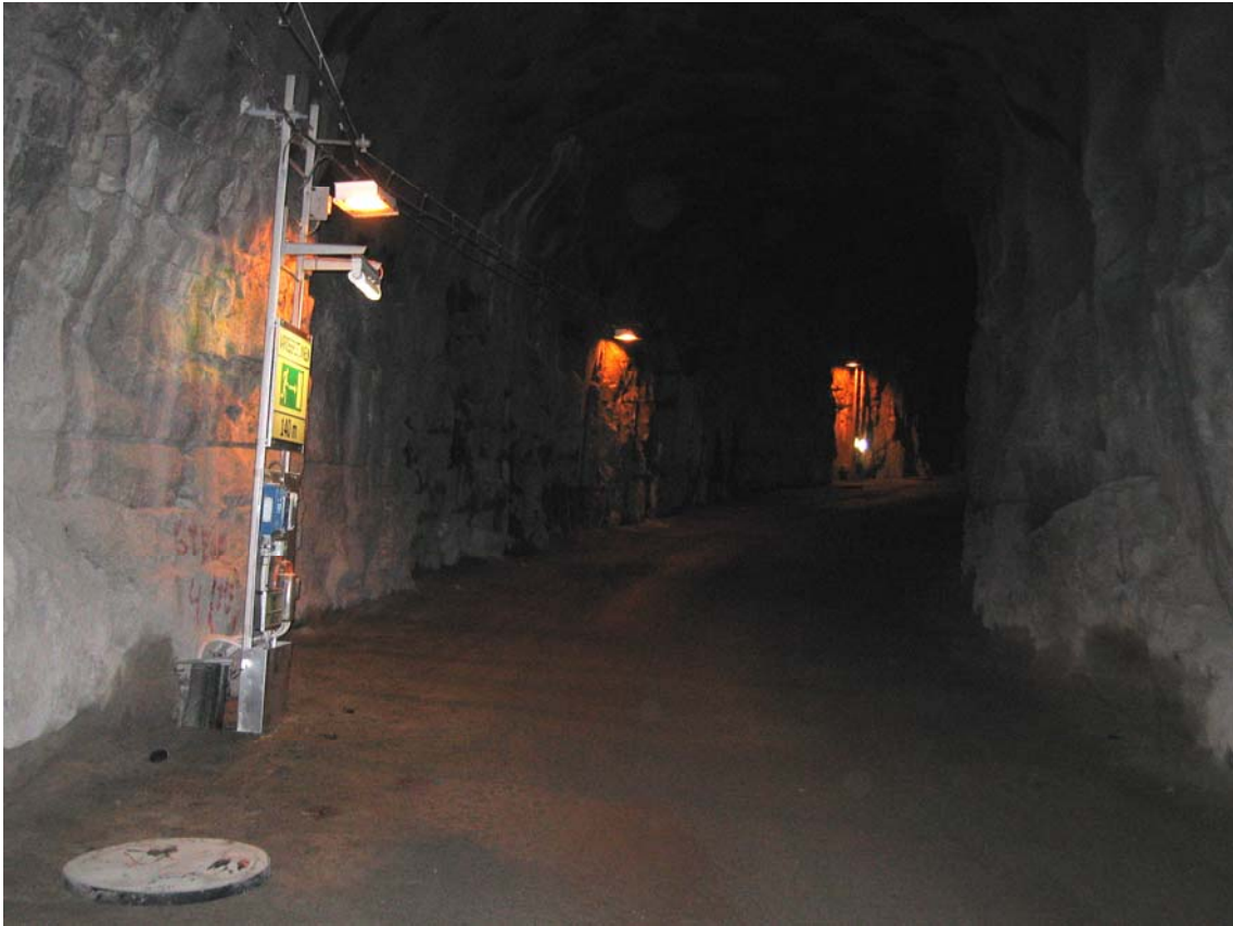
Figure 17 Example of an access tunnel.
