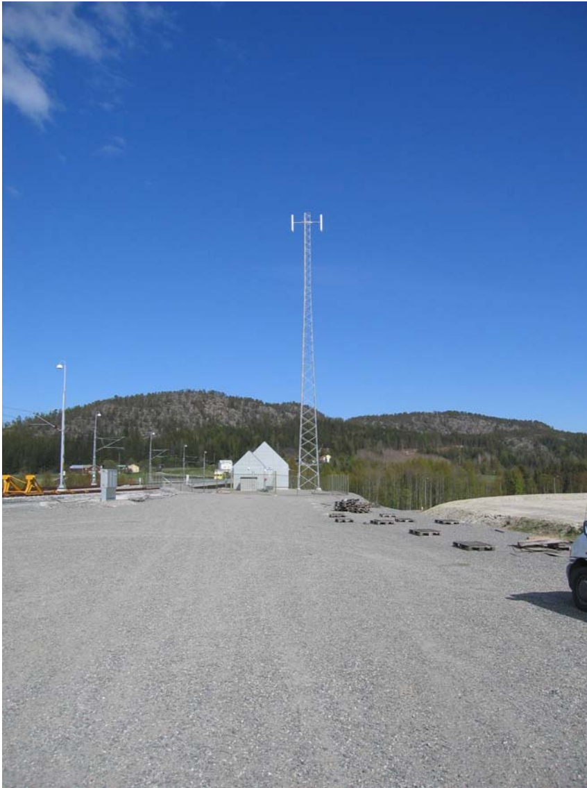
Figure 12 The picture shows houses for electronic equipment used for train operation control (signal and telecommunication). On the right a telecommunication tower is shown.
