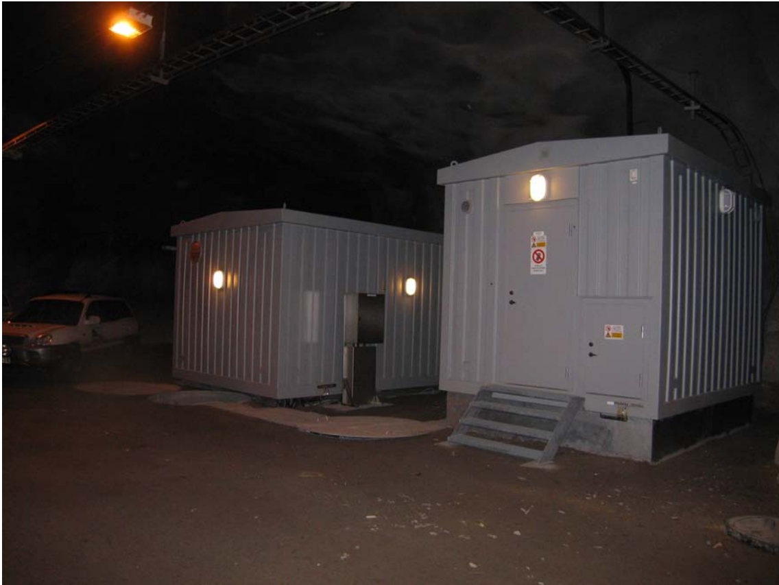
Figure 13 Houses for electronic equipments.
