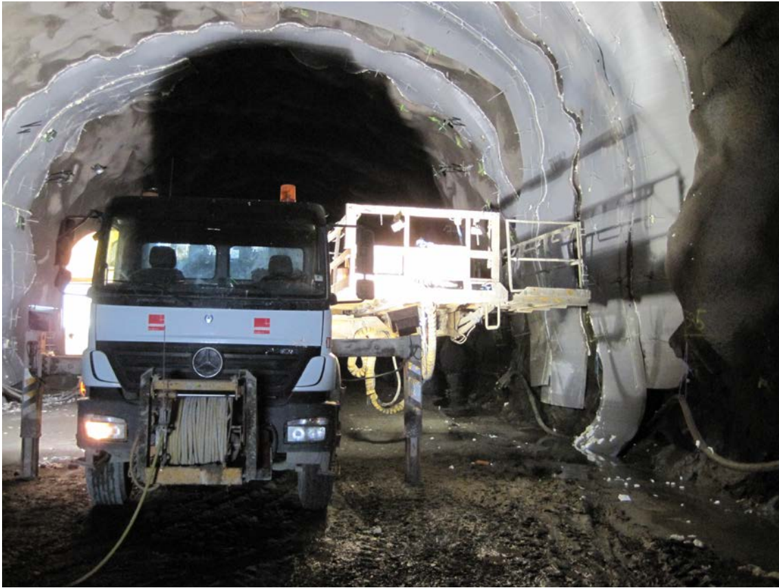
Figure 9 Lift for the assembly process of the standard drainage.
