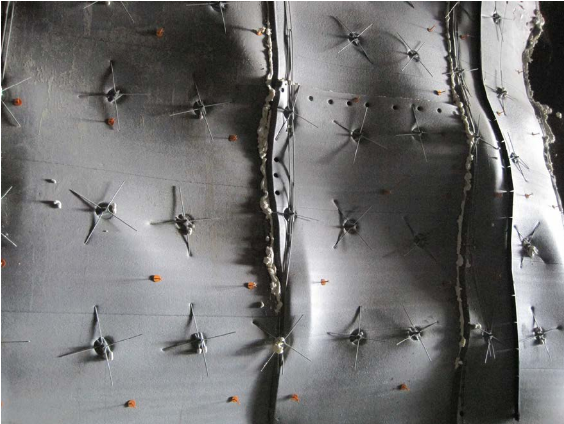
Figure 10 Mounted standard drainage ready to be covered with ordinary shotcrete.
