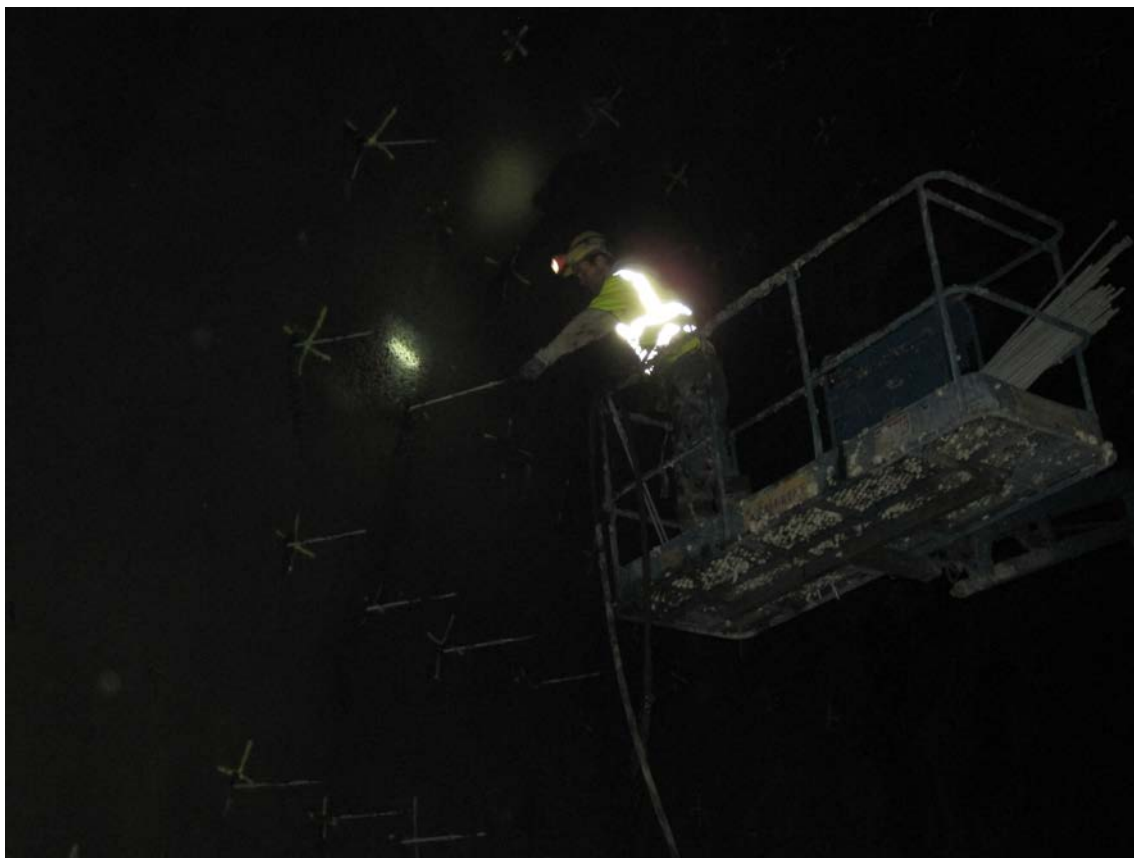
Figure 6 Mounting of threaded rods.
