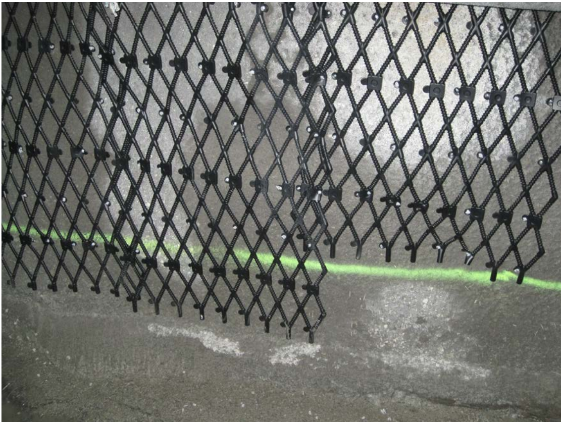
Figure 1 Mounted polyethene plastic lattice forming the drainage channels in the Rockdrain system.
