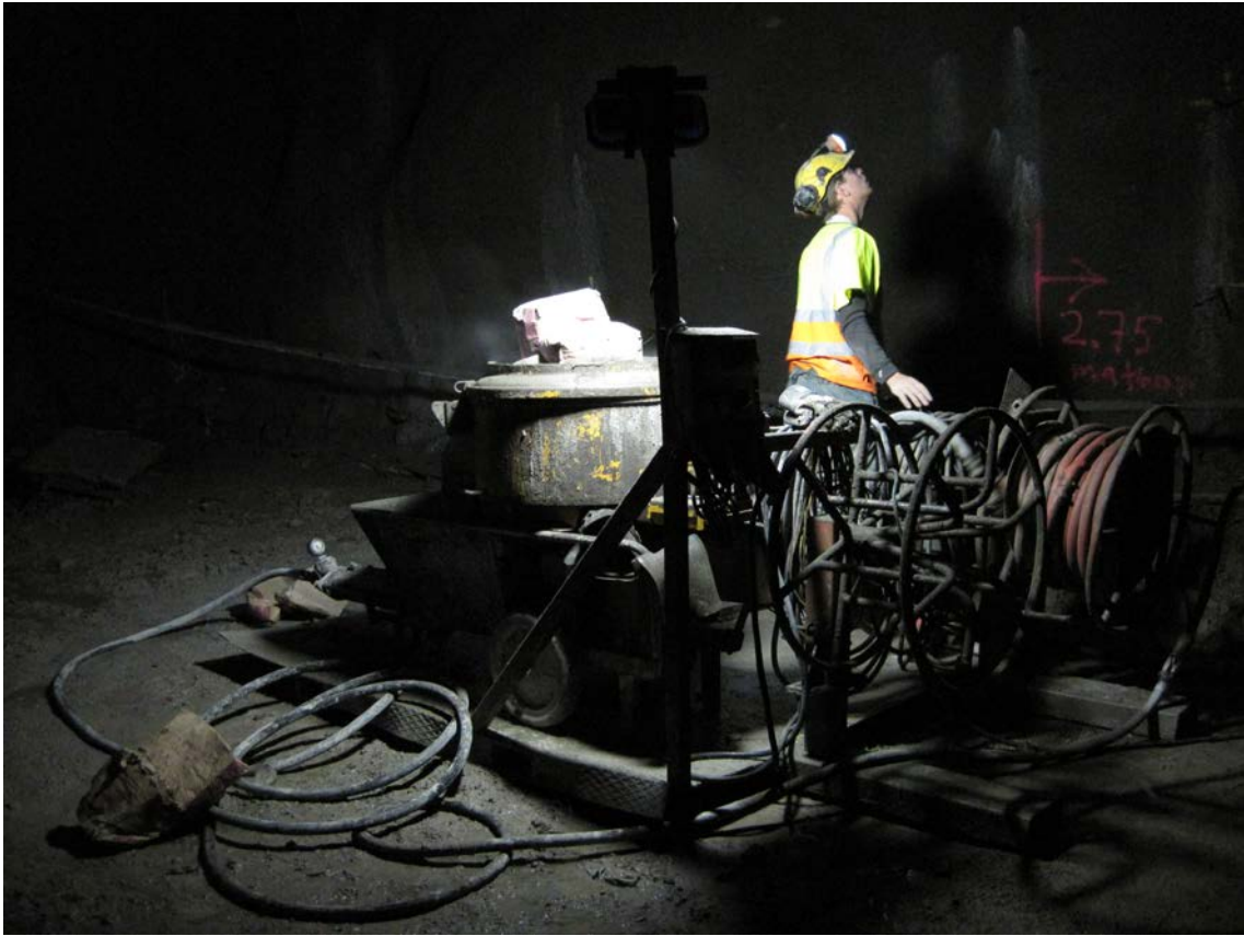
Figure 7 Mixing of cement paste for fixing of the threaded rods.
