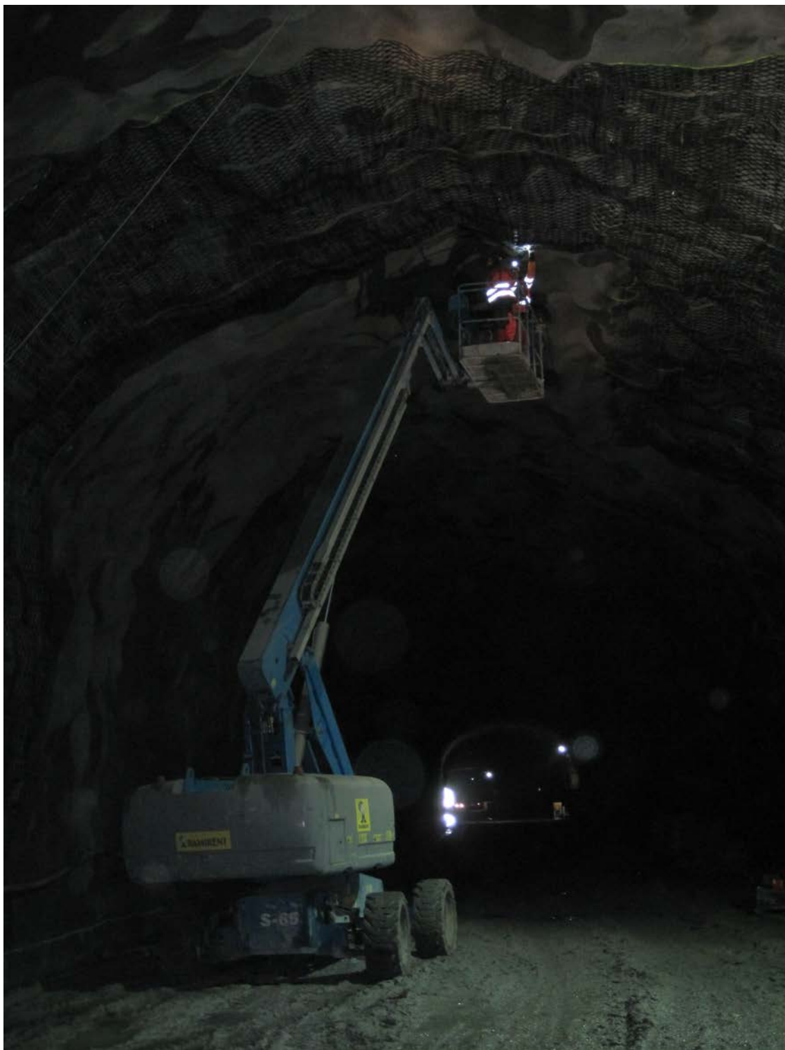
Figure 2 Mounting of the channel lattice using a boom lift.
